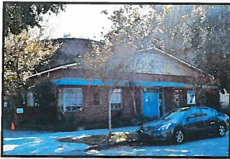
Figure 35. Cannon Street YMCA, 61 Cannon Street (Site #089-7843)
