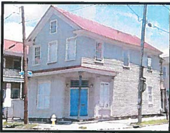
Figure 29. Corner store: 168 Smith Street, Site # 089-7876
