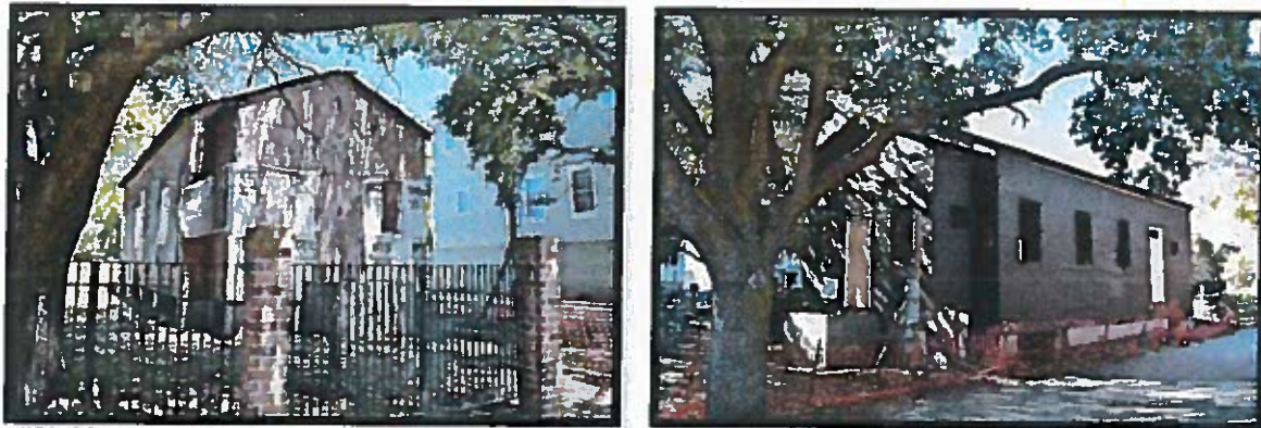
Figure 32. Chapel/Praise House: 78 Morris Street, Site #089-7900.
