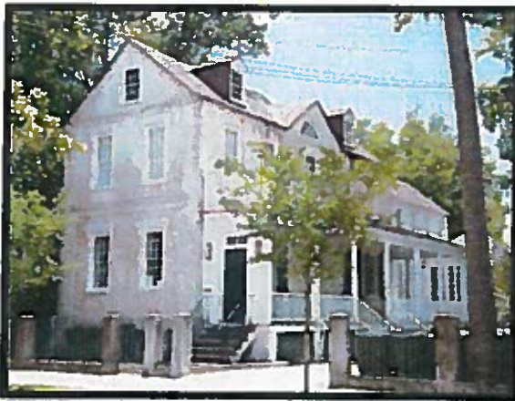
Figure 20. Charleston single house: 65 Cannon Street, Site #089-2109
