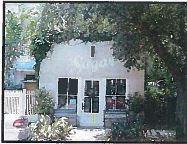
Figure 27. Enframed window wall: 59½ Cannon Street, Site #089-7841
