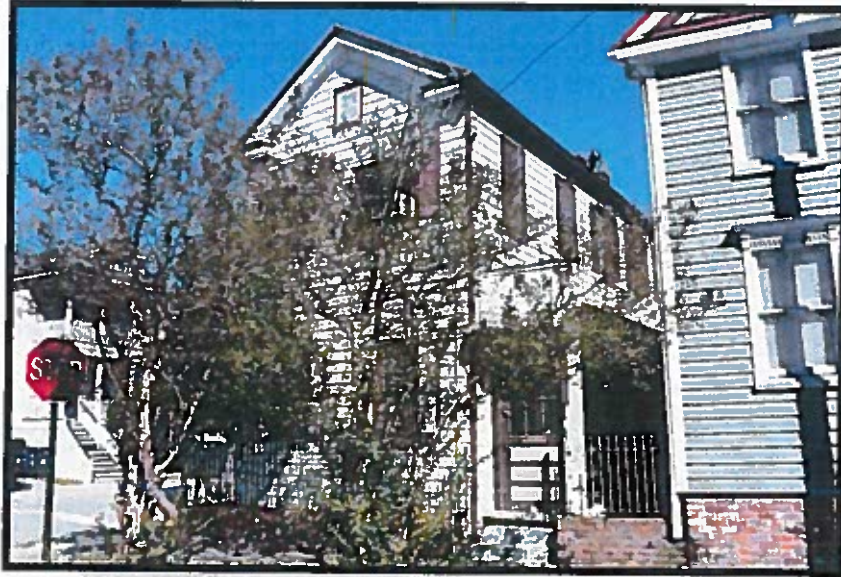
Figure 45. Lois A. Simms house, 28 Jasper Street (Site #089-7897)
